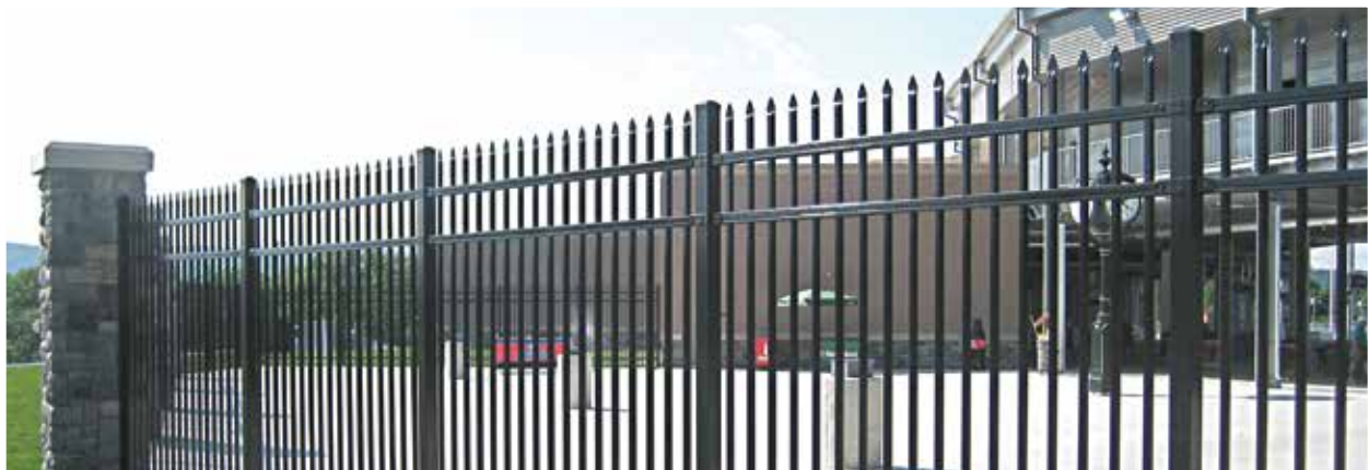
LIGHT INDUSTRIAL ORNAMENTAL STEEL FENCE
